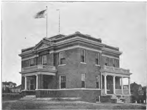
SIGNAL SERVICE ON WEATHER BUILDING, DODGE CITY.
